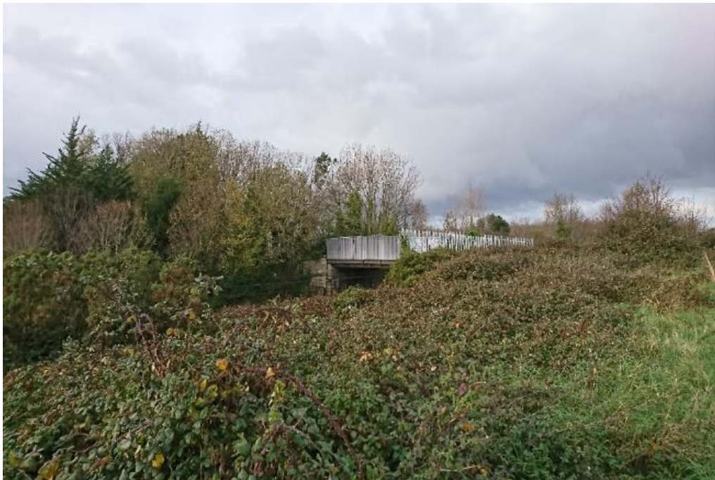
Plate 17.6: Bridge over DART tracks at Field 2.3, facing north-west.
