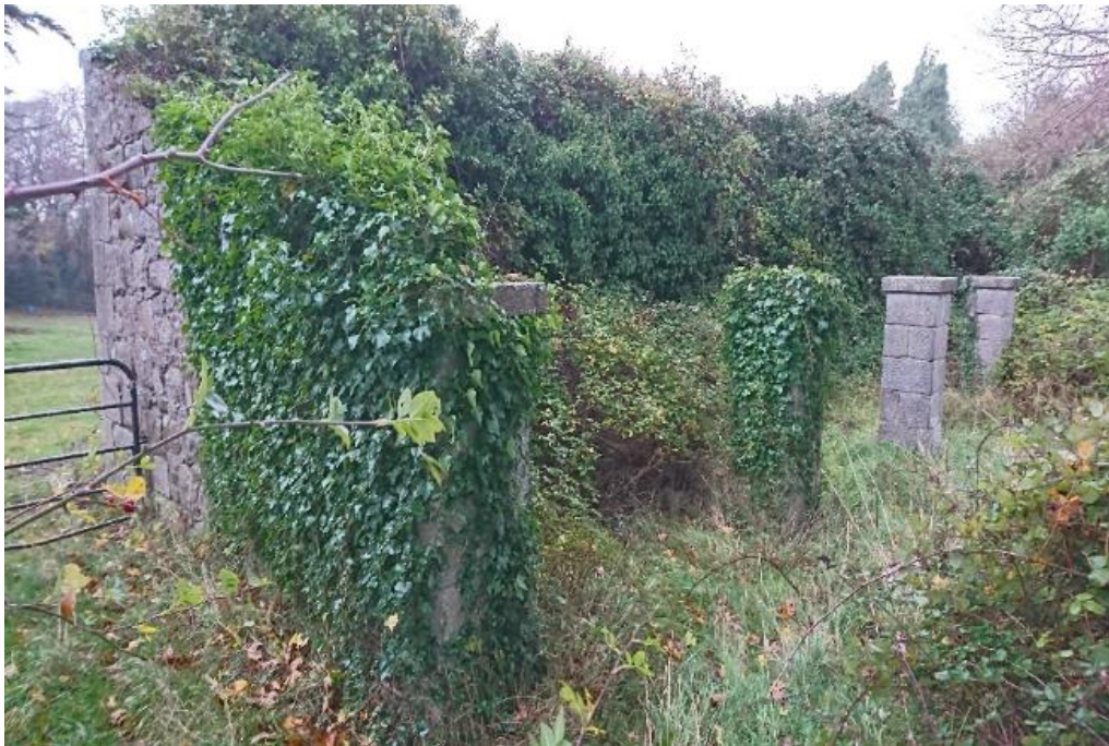
Plate 17.12: Rear walls of Corke Lodge in Field 3.3, facing south-west.
